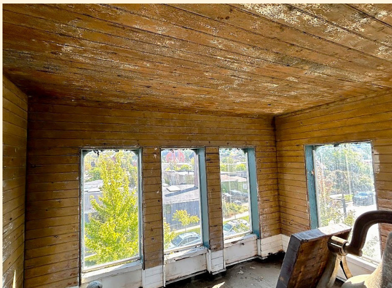
Bell Tower Interior
