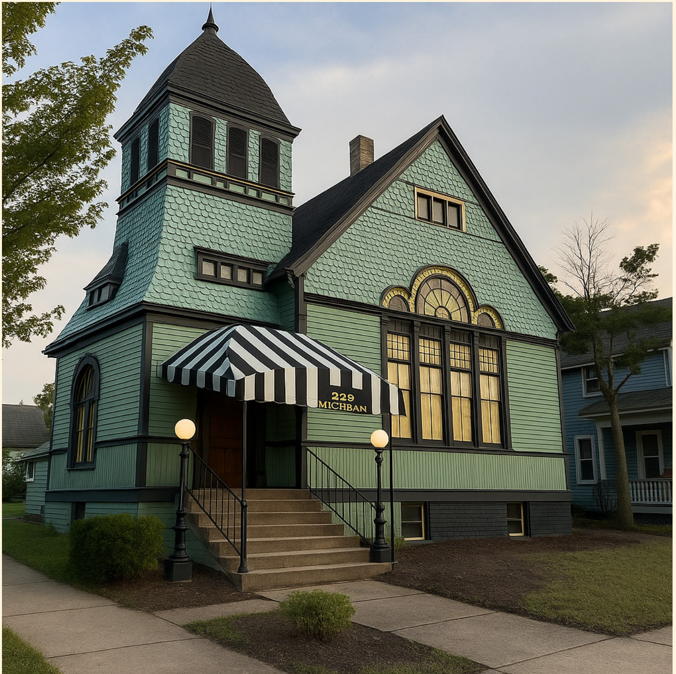
Rendering of the building once exterior restoration work is finished. Final colors have not been selected.
